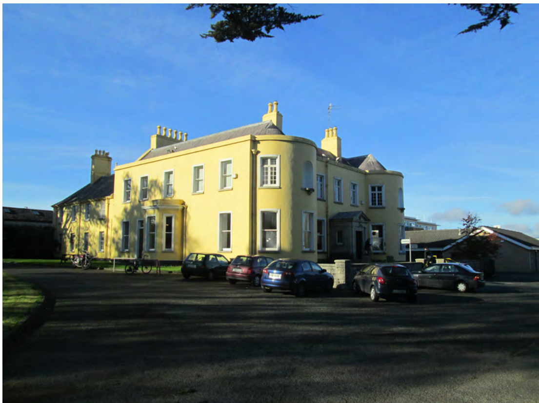
Figure 11.1 Burton Hall, Arena Road, Sandyford
